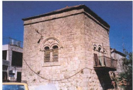
Two-storey house, Al-Birch city
